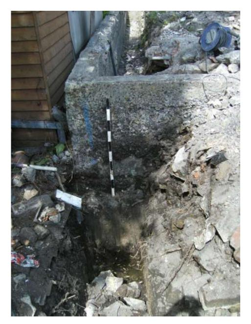
Plate 5. Depth of foundation trench
