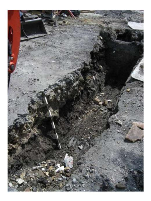
Plate 7. Depth of foundation trench
